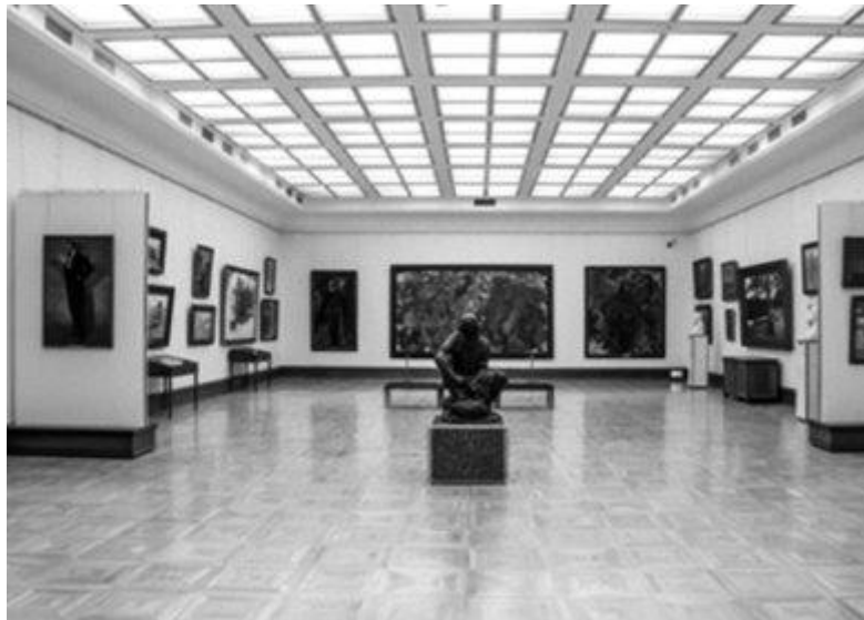
Fig. 1. Use of light-diffusing glass in the exhibition hall of the Tretyakov Gallery
